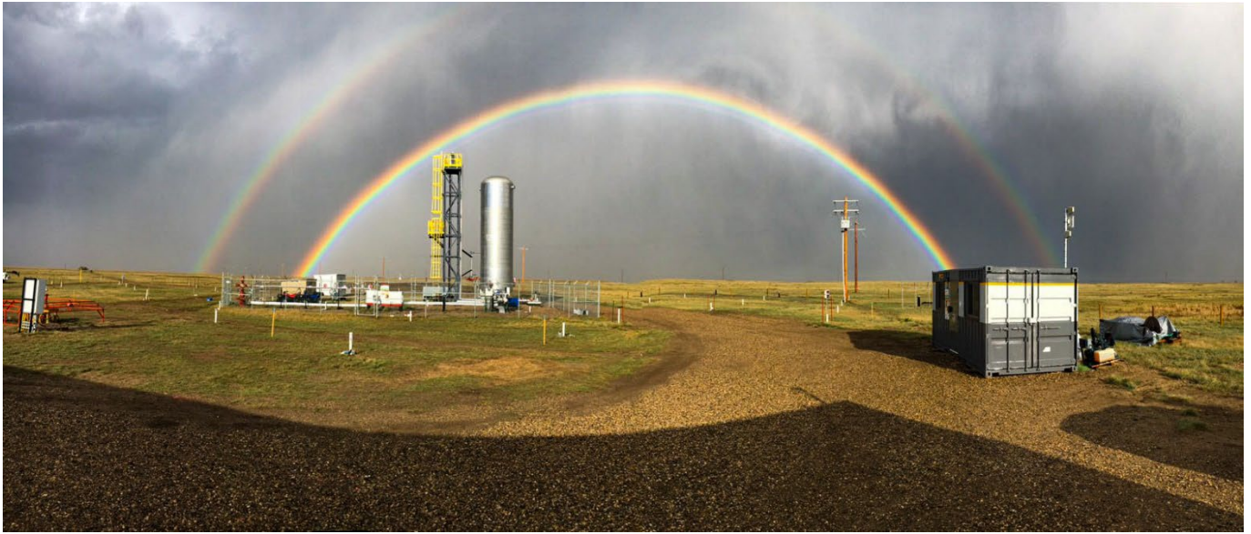
Figure 1: Carbon Management Canada (CMC) Newell County Facility in Alberta, Canada (Image courtesy of Maurice Shevalier).
