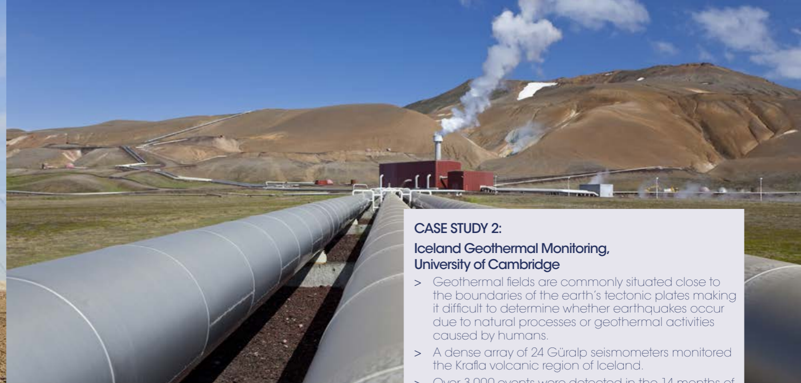
IMAGE 2: KRAFLA GEOTHERMAL POWER PLANT, ICELAND
